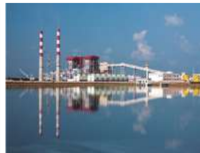
Matarbari Power Plant Total Cost USD 4.40 Billion Commencement 2014 Estimated Completion 2024
