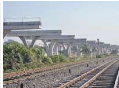
Dhaka Elevated Expressway Total Cost USD 1.63 Billion Commencement 2011 Estimated Completion 2022
